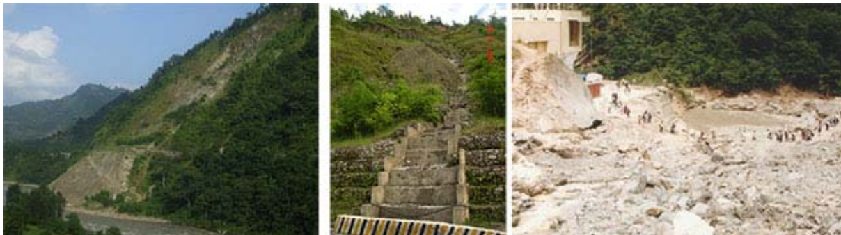
Landslides and their mitigation in Kathmandu-Pokhara road section
