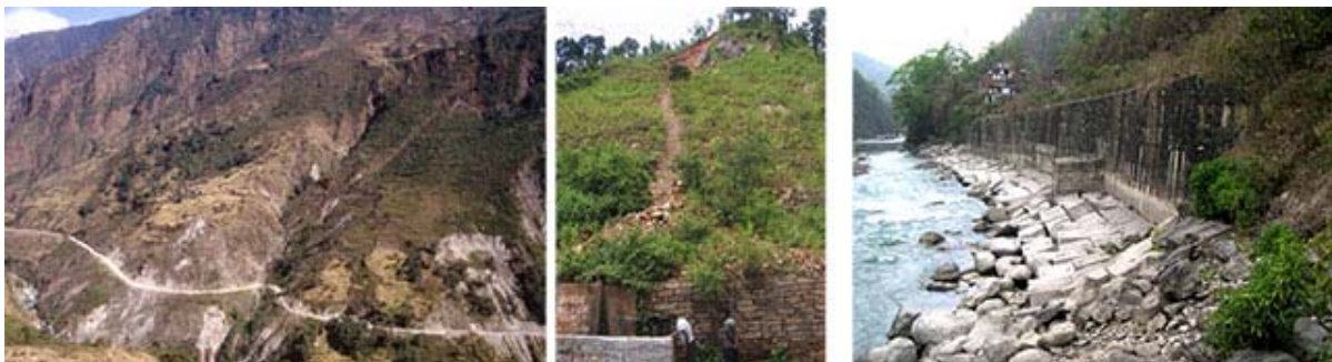
Geo-disasters and their mitigation in Kathmandu-Kodari road section
