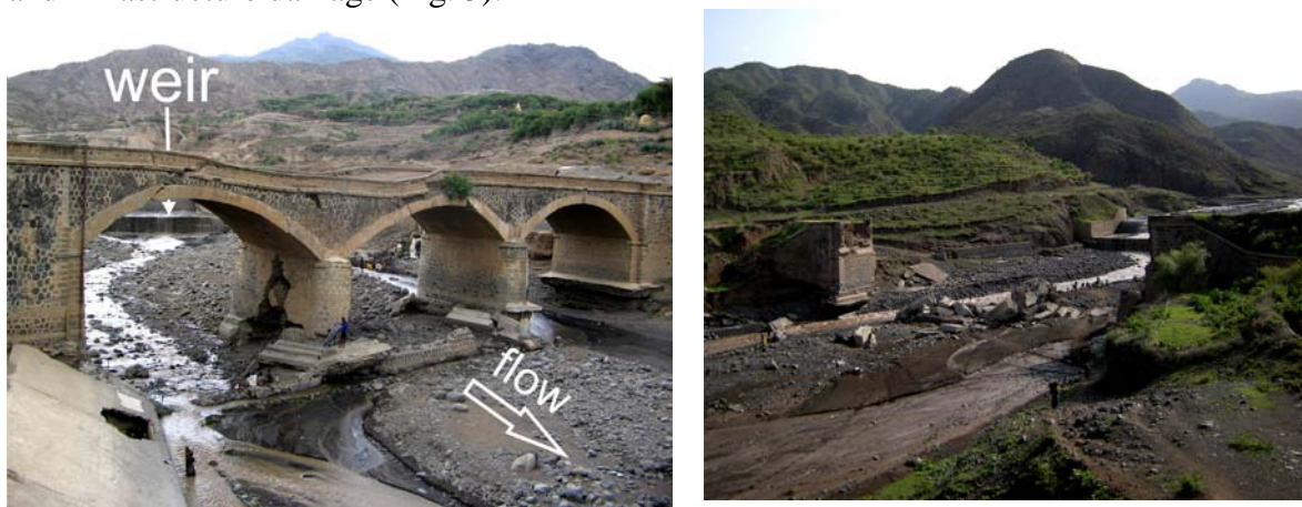
Fig. 5. The Golina R. bridge on the Woldya-Alamata road in 2006 (left) and after the ultimate collapse in 2008 (right) (Billi, 2011b).
