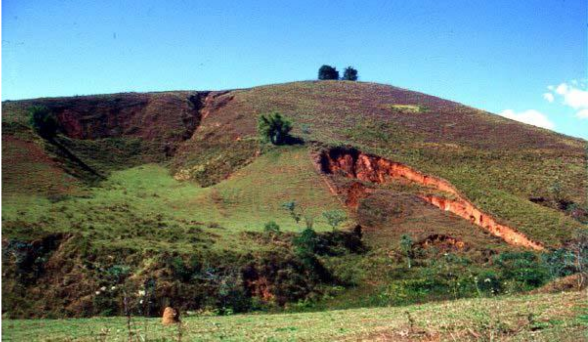
BRA 3/46: Reduction of strength of rock due to deeply penetrating weathering enhances susceptibility of slopes to landsliding. This photograph was taken on the road going from Bananal westwards and shows two landslides of different ages. The one on the right is a good example of slump and, judging from the very fresh appearance of the rear scarp, is very recent. To the left is the scar of an older landslide, partly vegetated but also subjected to shallow translational sliding and gullying. The landslide mass has now a smooth evened surface and the form approaches the depositional 'rampa' stage. Low earth mound in the foreground testifies to the important role played by soil organisms in forming the structure of the superficial layer.
