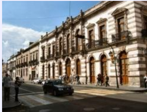
Photo 2 Architectural heritage of Morelia.
