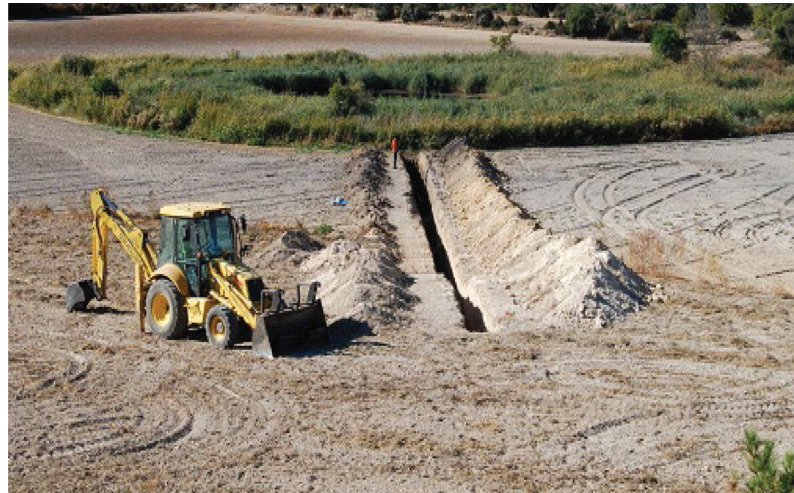
Trenching investigation in paleolakes associated with tufa mounds, Pyrenees
