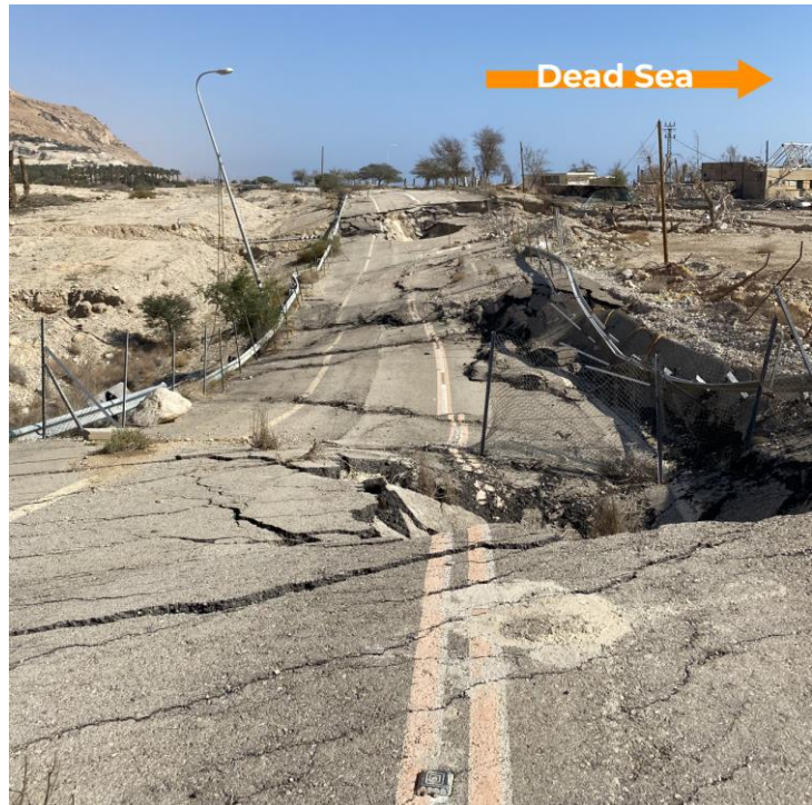
Figure 4. Sinkholes affecting old highway.
