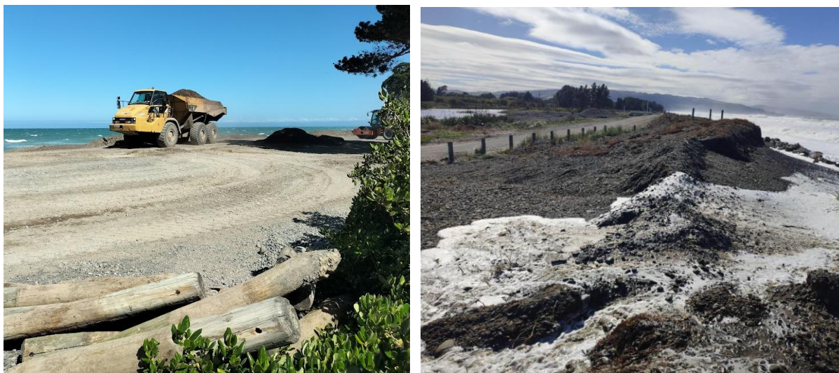
Figure 36. (Left) Bund reconstruction at Amberley Beach and (right) water washing over bund. Images from: S. McSweeney and Hurunui District Council (2023).
