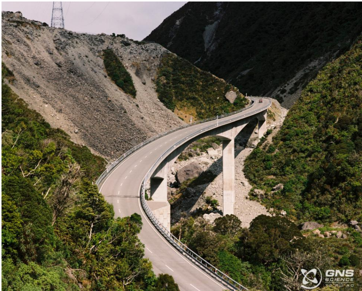
Figure 17 – The Otira Viaduct, looking up valley. Note the large boulders in the stream bed, and the exposure on the left of the rock avalanche debris. Photo: D. L. Homer.
