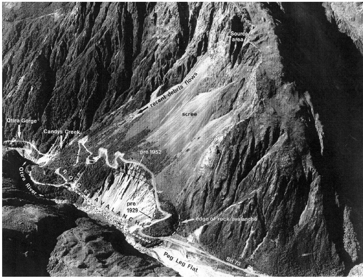
Figure 17– View of the original road alignment, and planned alignment of the viaduct at Otira Gorge. The source area of the major rock slope failure is demarked, along with other key features. Annotated photo reproduced from Billings (2004), photo originally taken by D. L. Homer.
